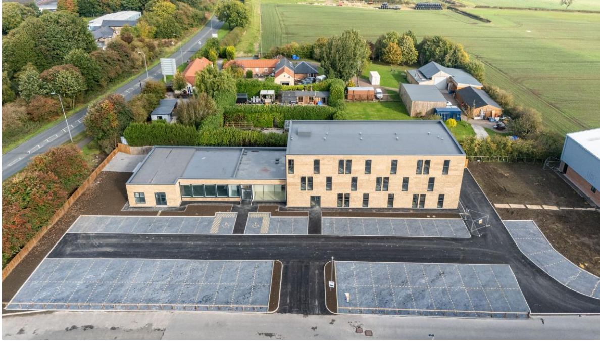
Completed finish in adjacent office
